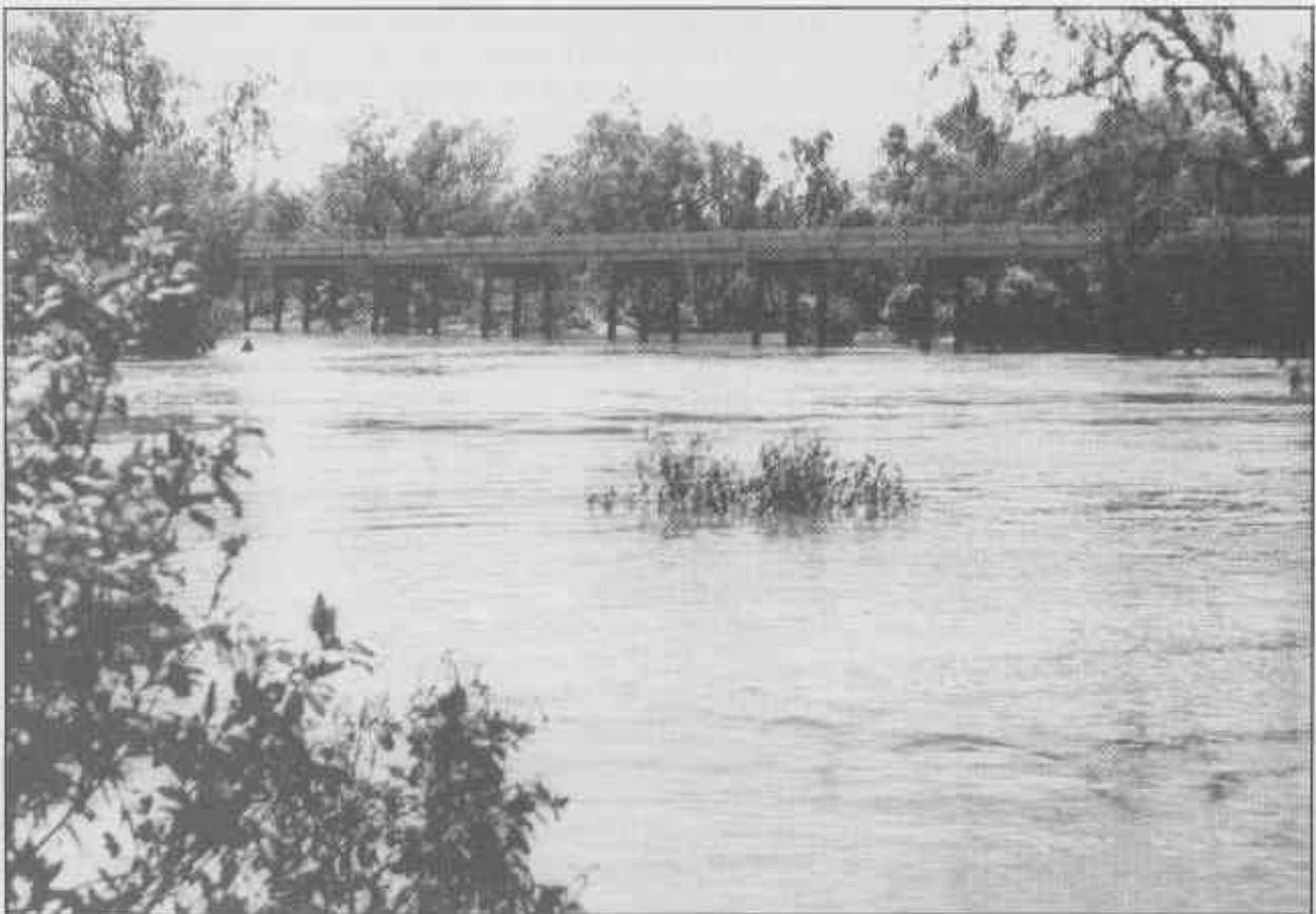
Fitzroy River - late March, in flood. Willare Bridge in background.
