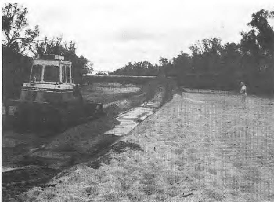
Sand Excavation Burlong Pool
