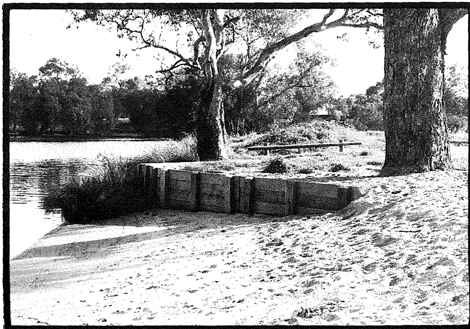
PLATE 14: Foreshore works to protect vegetation, Bassendean
