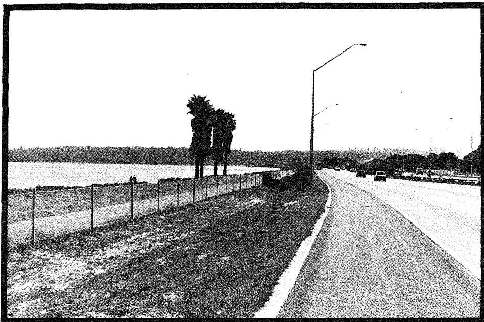
PLATE 15: Access to the foreshore has been restricted due to the Kwinana Freeway
