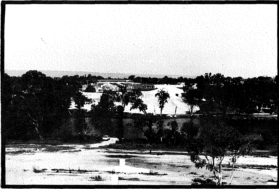
PLATE 10: Earthworks for the Redcliffe Bridge, due for completion 1986/87
