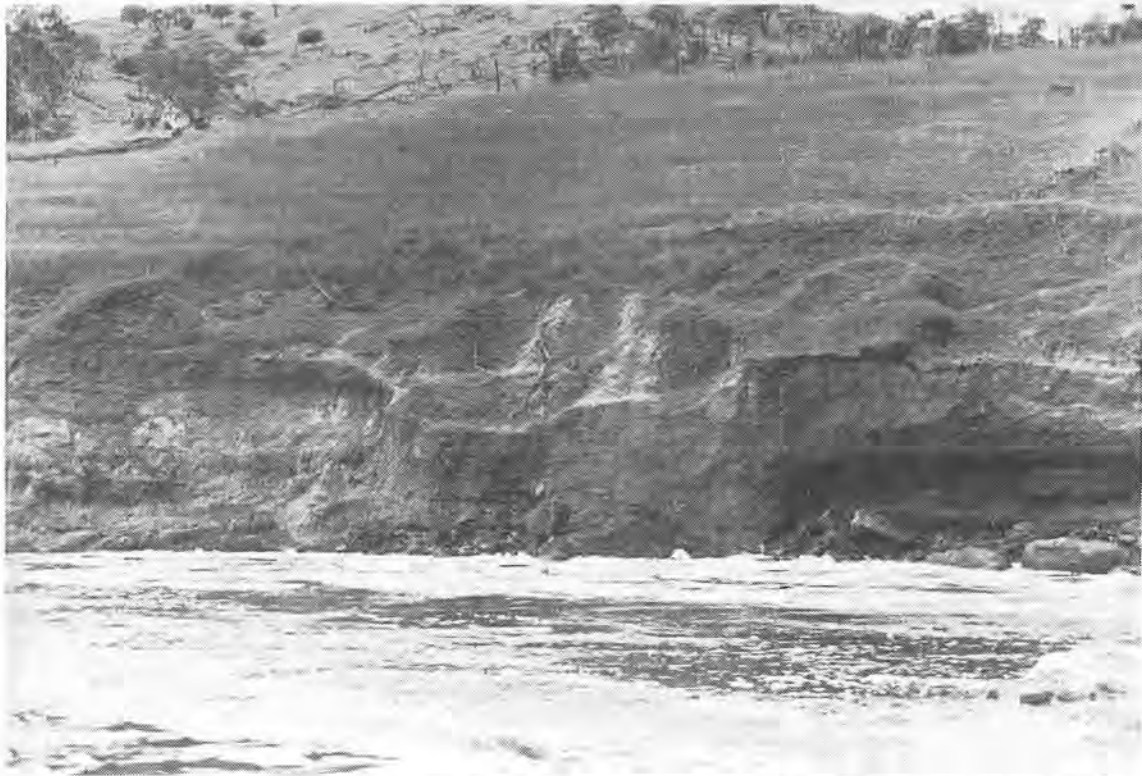
River bank erosion is occurring along the Avon River as a consequence of the clearing of foreshore vegetation, the grazing of stock on river banks and uncontrolled public access
