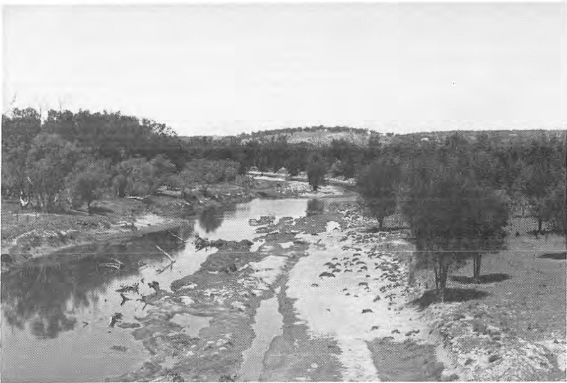
The River Training Scheme has had an effected on the process of siltation within the Avon River
