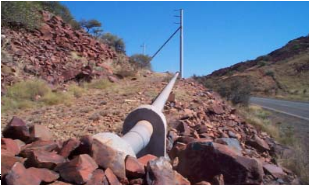
Plate 7-1 View of the existing water pipeline within the Hearson Village Road Reserve, looking west.
