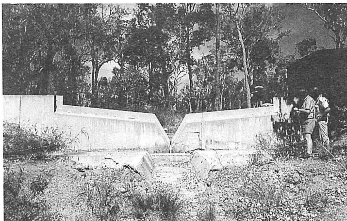
3.2 Downstream of weir. This weir has been designed to never drown out and obviously fish could never bypass the control structure.
