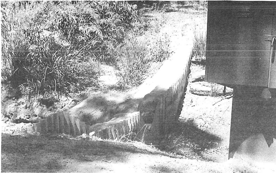
1.1 Weir during summer (February 1987)
