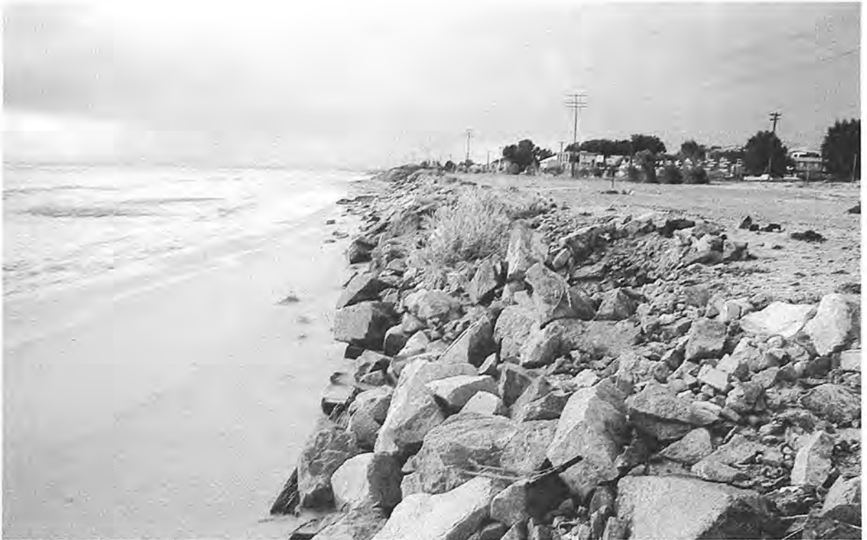
Photo 10 Railway Reserve - rock wall and backing level land
