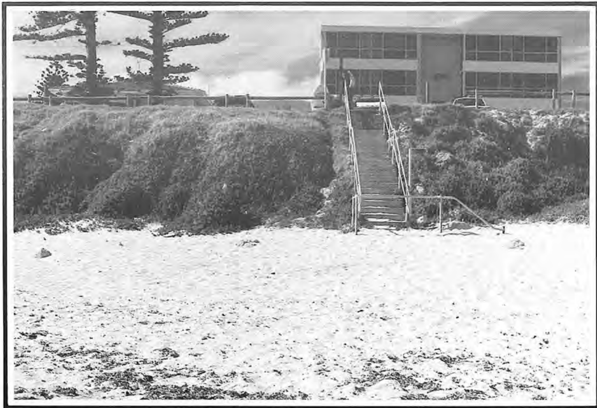
Photograph 10. Concrete steps at Deane Street. Storm water reaches them during winter. Solid steps should not be built so close to the water in the future.
