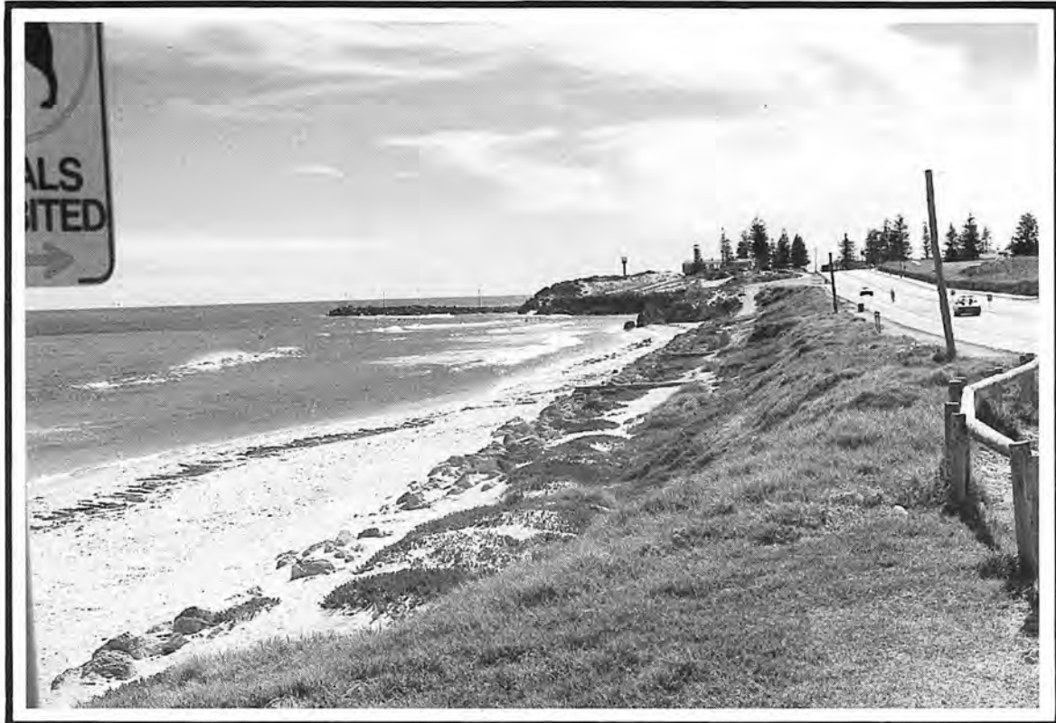
Photograph 12: Storm water pipes near Mudurup Rocks. A post and rail fence is recommended along the dual use path to protect pedestrians from traffic on Marine Parade.
