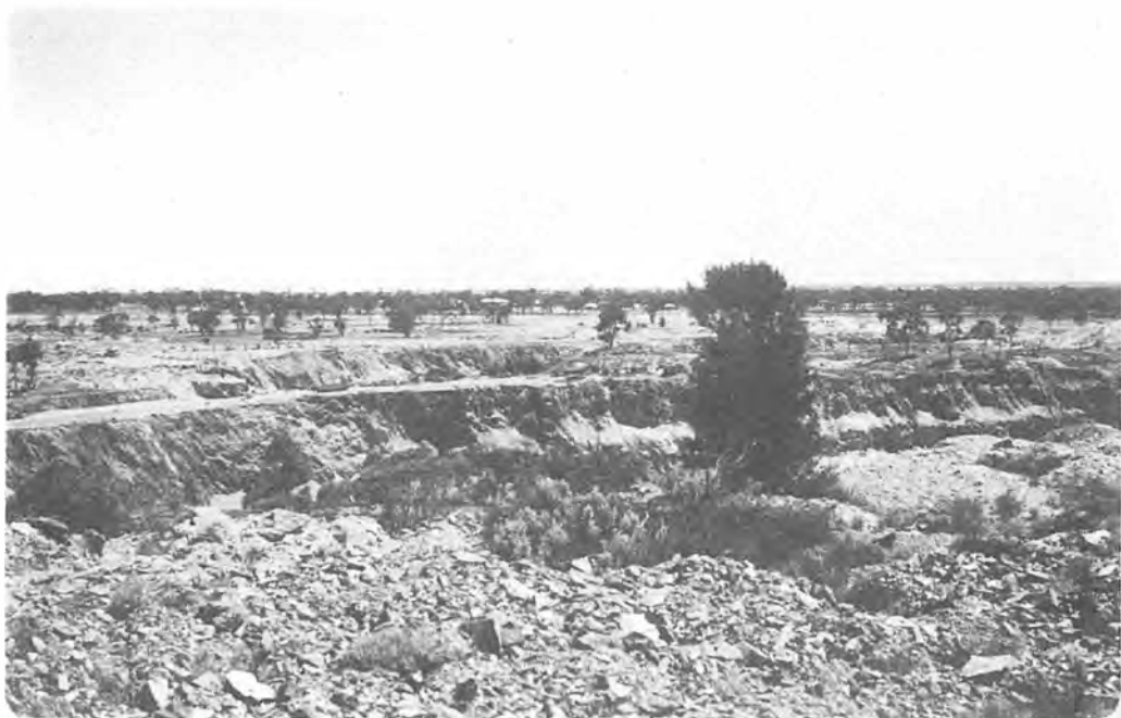
PLATE 22 The Great Western open cut and adjacent mullock dumps.
