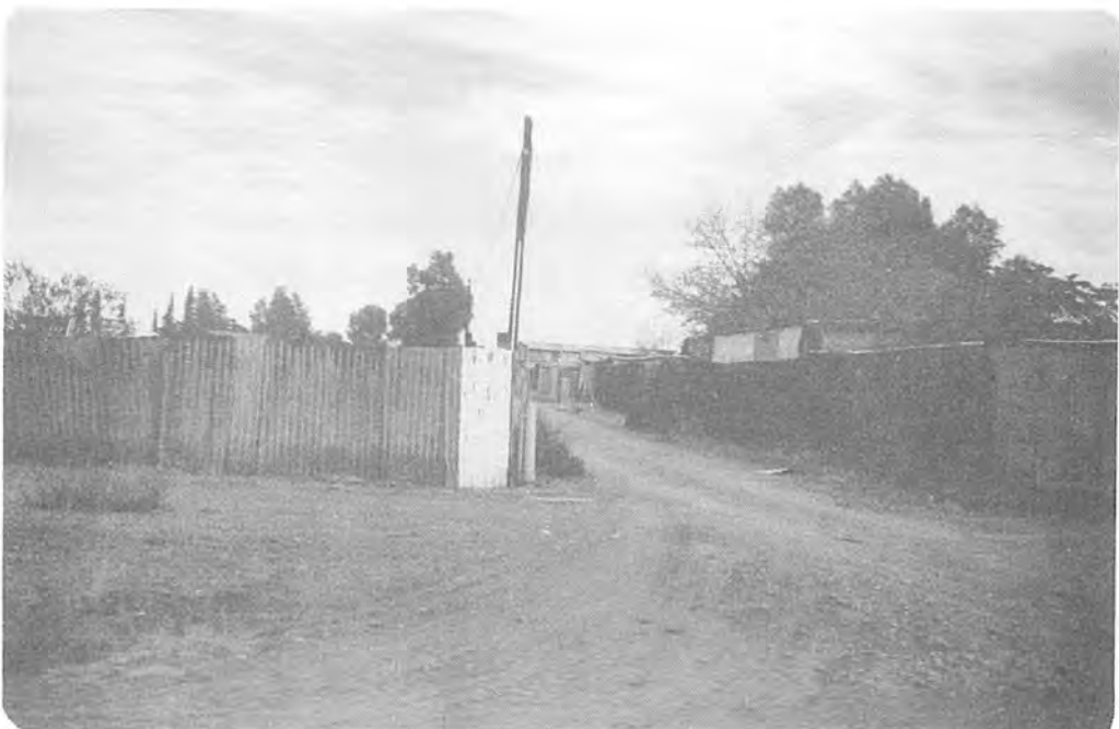
PLATE 4 Unsealed service lane-way in Kalgoorlie.
