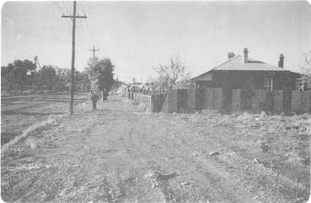
PLATE 3 Bare road verge within the Kalgoorlie townsite.
