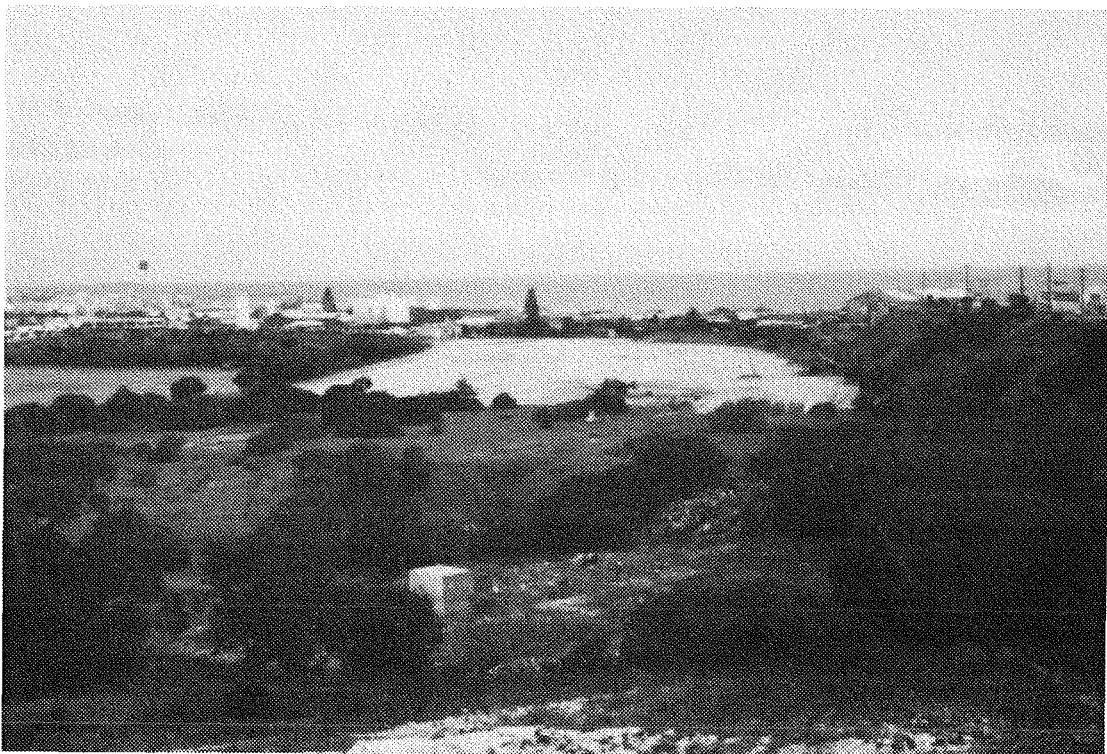
Plate 7: CSBP Hill west across IFAP ruins and CSBP site to Rocky Bay, cleared SEW site, North Fremantle industry and Indian Ocean.
