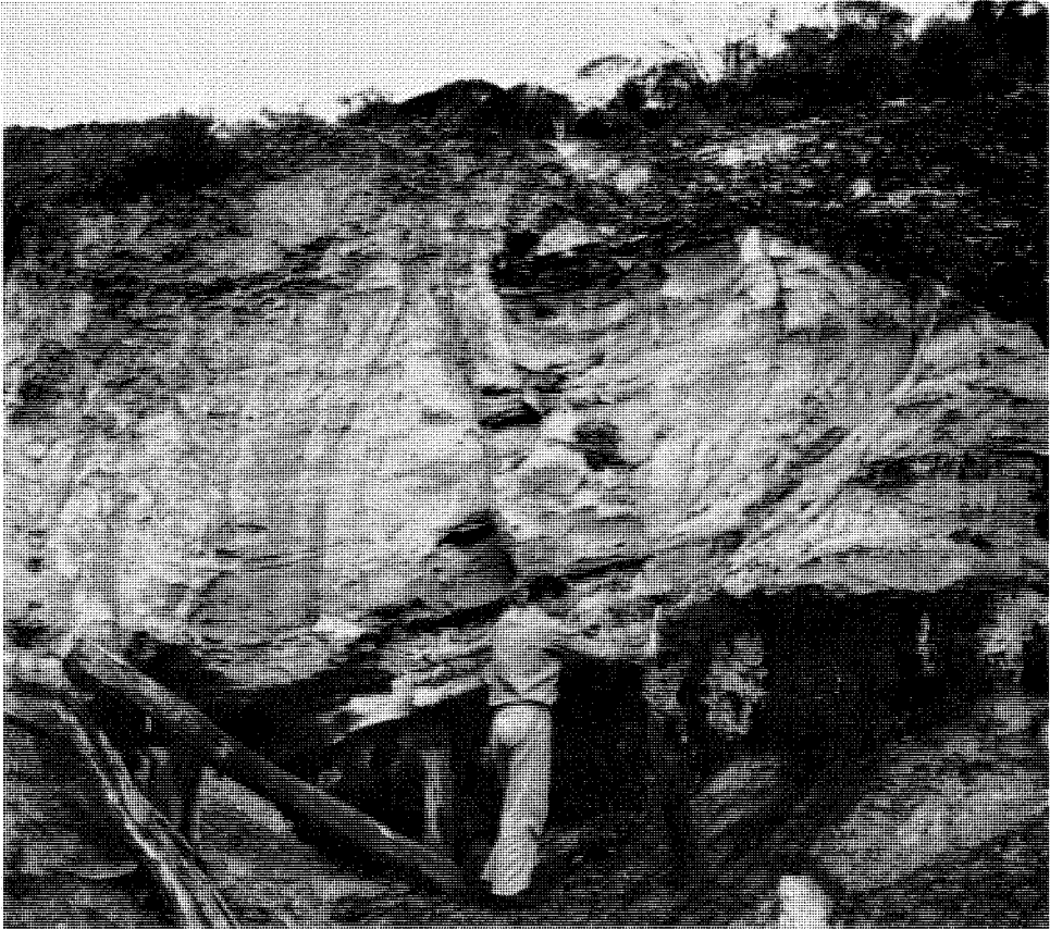
Figure 24. Adit driven along a coal seam in the Irwin River Coal Measures on the North Branch of the Irwin River.
