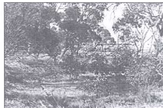
B. Roadworks had left a hollow - bingol. Young trees! (P. Hussey)
