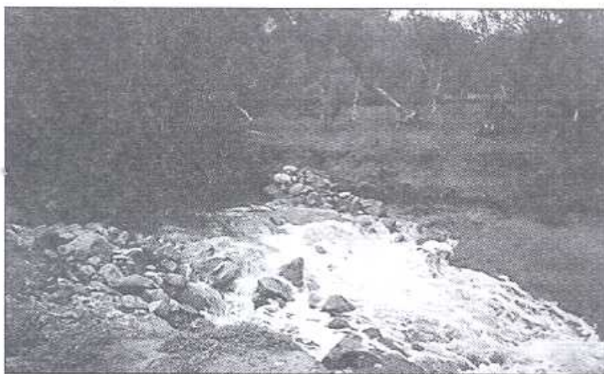
A rock riffle as built on Spencers Brook.
