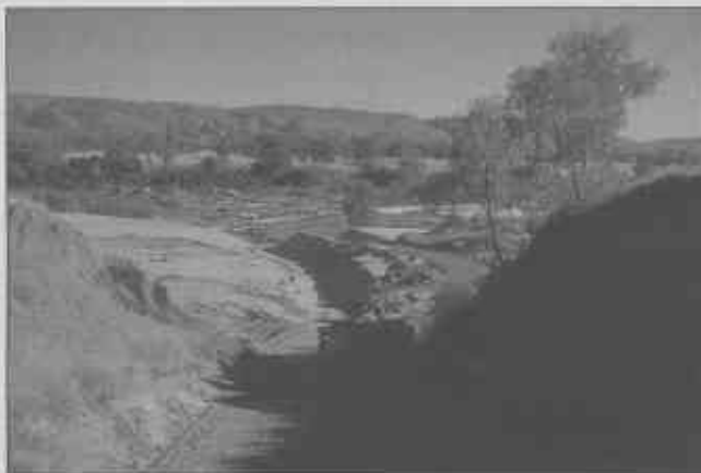
Ivanhoe Crossing, June 1953. Prior to construction of the dams upstream, the river was subject to huge floods in the wet season and dried back to pools during the dry season. Note the large sand bar which was deposited across the approach to 'the crossing' in the 1952/53 wet season. Photographer: W.A.C.Wright.
