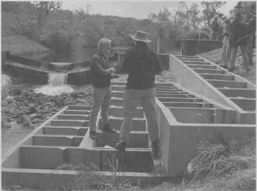
Alan Danks (Regional Leader Nature Conservation, CALM) and Steve Janicke (Rivercare Officer, Department of Environment) standing on the fish ladder with the weir in the background
