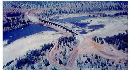
Building the Diversion Dam, 1962 Photo: unknown
