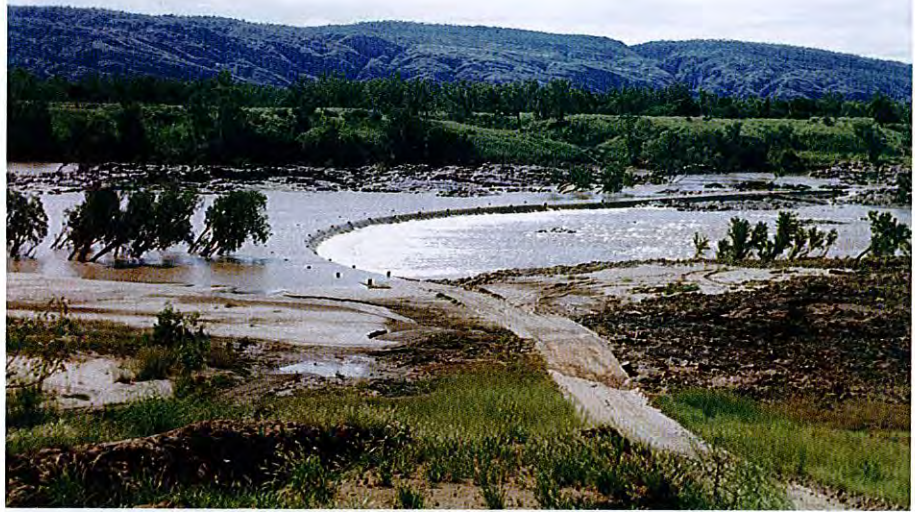
Ivanhoe Crossing in the 1960s, showing a sandbank deposited over the road and paperbarks growing upstream on a rocky shelf in the water. Photo: Barrett
