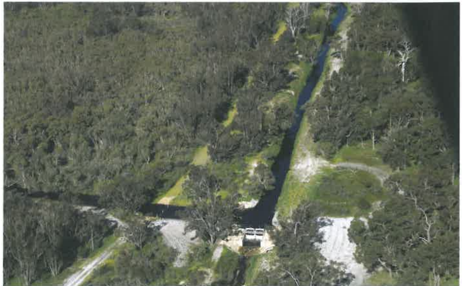
Aerial view of Mealup Main Drain, August 2012, showing diversion weir in operation Photo: Ross Rose
