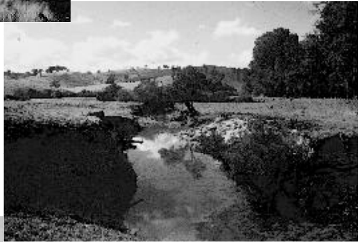
Plate 14: D1 grade foreshore. Subsidence and undercutting are commonplace, but vegetation still supports some sections of foreshore (i.e. shrub in right foreground, steep grassed embankment on left foreshore, small tree in right middleground and upstream. (Photo by Peter Williams).
