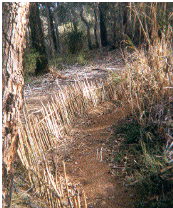
Giant reed, dried for a minimum of 2 years, used as brush fencing to prevent erosion.
