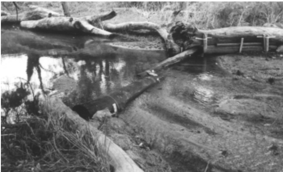
Plate 5: Large woody debris riffle built on the South Dandalup River, Pinjarra (WA).
