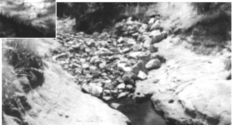
Plate 3: Riffle built on Spencers Brook.
