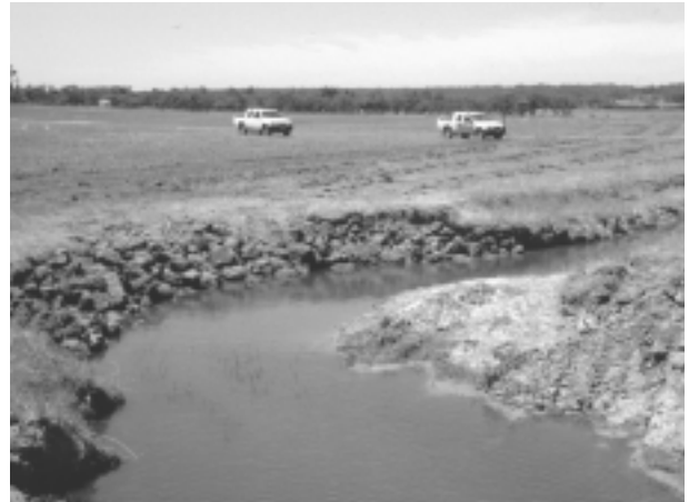
Figure 22. Bank armouring. Note that armouring a bend with rock, for low flows, may aggravate turbulence and erosion during high flows.
