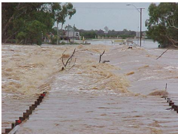
Figure 21. Flood flow in Gascoyne River at the old Nine Mile Bridge – March 2000.
