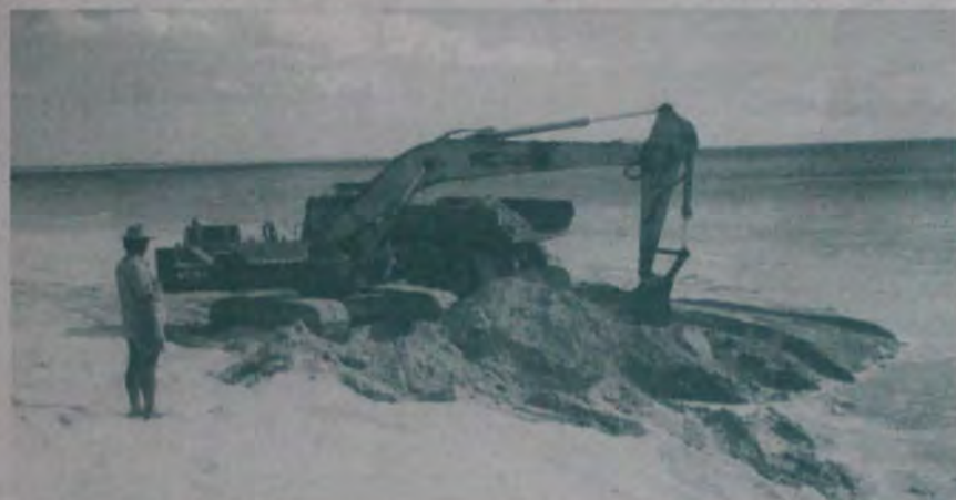
Jeff Anderton supervising the removal of the groyne at Port Kennedy.
