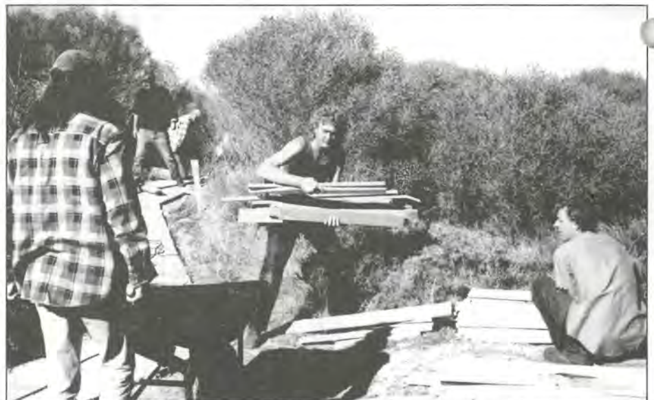
Volunteers Paul Bunce, Glenn Smith, Paul Cross, Greg Verboon and Misha Kalkowski work on the new "Bushucker Trail" being created at Navagebup. This Learning Centre on bush foods and medicines has been funded by WMC Resources Ltd.
