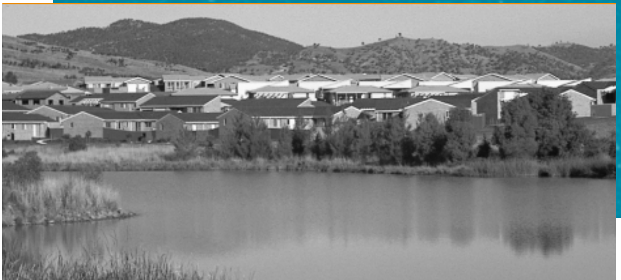
Stranger Pond (Isabella Plains, ACT), providing an important pollution control facility protecting the Murrumbidgee River, as well as enhancement of landscape and recreational values.
