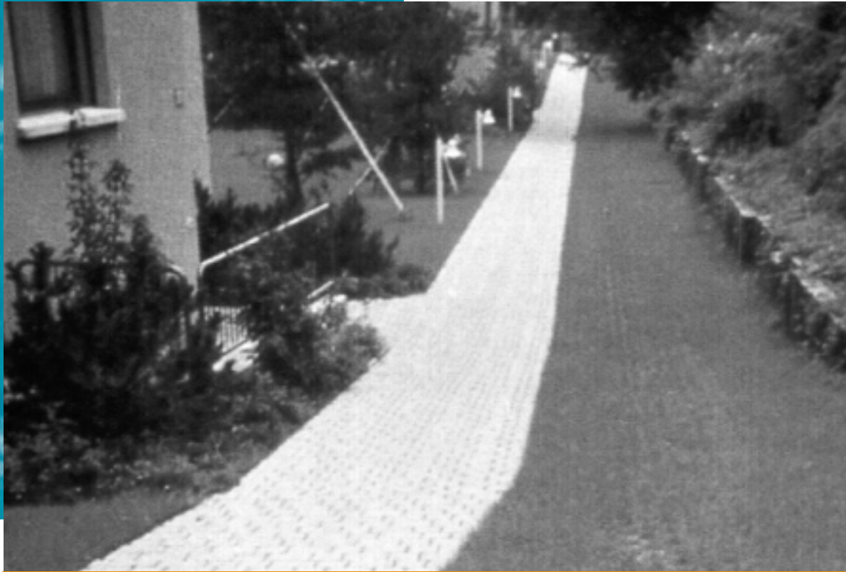
Integrated drainage and landscape: use of porous pavement on right to form a drainage swale. Photo: Peter Michel
