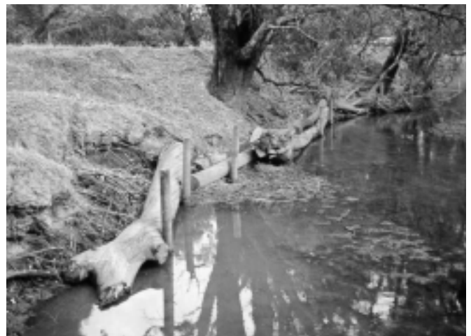
Logs pinned against bank.
