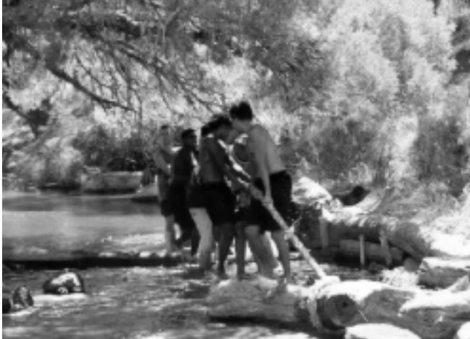
Installing logs at Fairbridge site.
