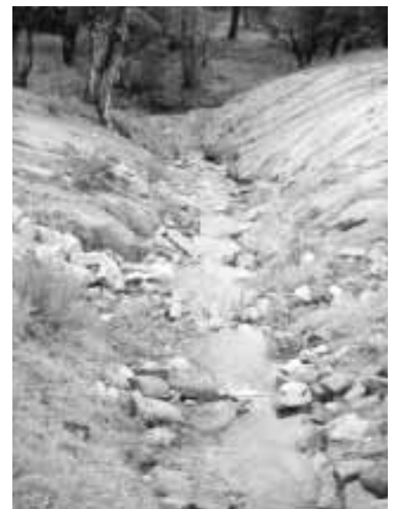
Figure 4. Rock riffles and matting installed on Southernwood Creek.
