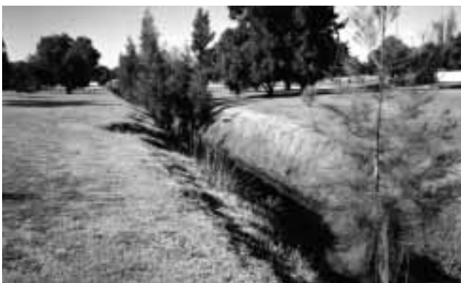
Figure 14. Bannister Creek prior to restoration works.
