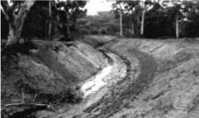
Figure 18. Rock gabions used to stabilise the outer bank.
