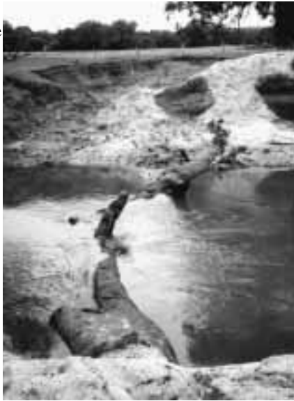
Figure 7. The riffles were constructed with the root balls of the logs buried into the bank to anchor the logs and the tapered ends pointing slightly upstream. A scour pool has formed in the centre of the channel.
