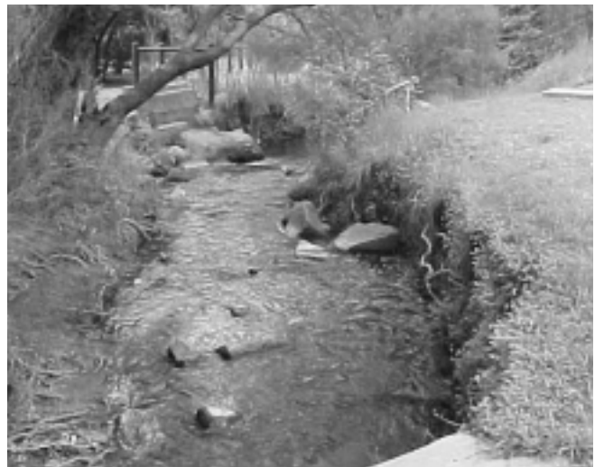
Figure 4. Bank erosion. This site is on the Neerigen Brook in Armadale. There is severe erosion on the right bank and rock gabions are planned for this site.
