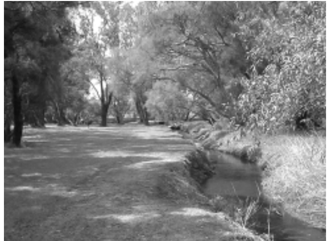
Figure 3. Bank battering site. Located near Corriedale Place in Thornlie only 100m from the Canning River which has spiritual significance to the local Aboriginal community. Erosion was causing the stream banks to slump and the stream is slowly getting wider. Battering to a 1:4 slope and jutemat, to stop erosion of the sandy soils, will be used in the rehabilitation of the stream banks.
