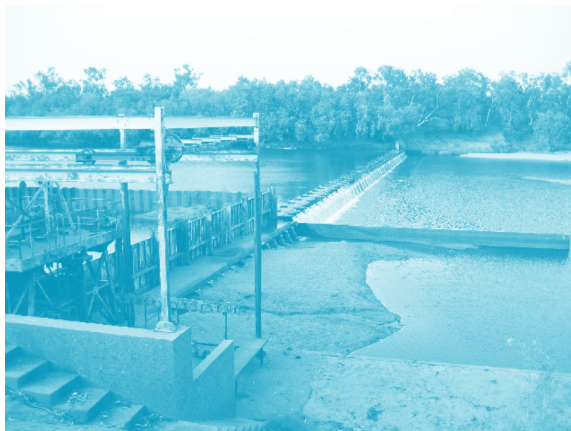
The Barrage at Camballin
