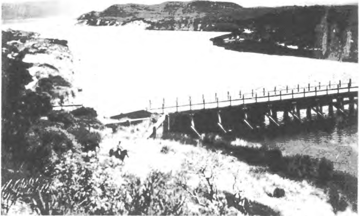
Torbay Inlet barrage and floodgates, built 1912. Photo: A. Shirley.
