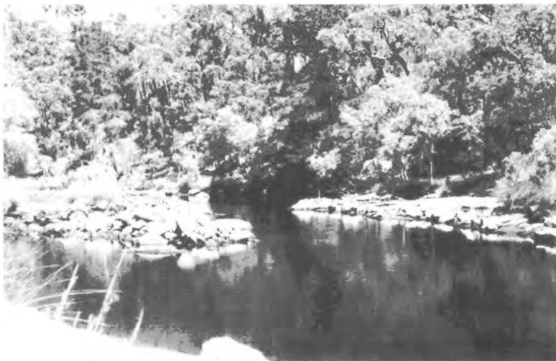
Channel blasted through the rock bar in the Kalgan River.
