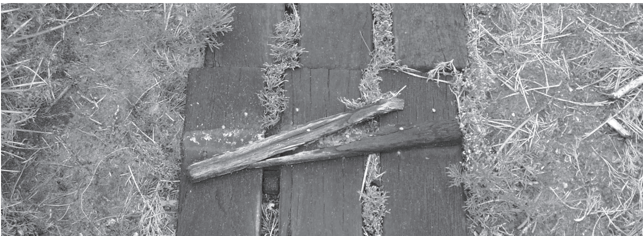
Figure 10. A charred board-walk with split cross tread and protruding nails, moderate-poor condition but moderate-excellent / excellent effectiveness rating for Bibbulmun Track in WCHNP
