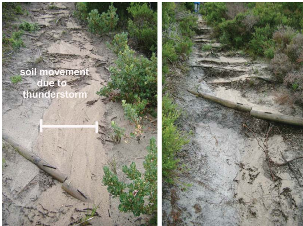
Figure 17 Ineffective water bars on the Peak Head trail, suffering from a lack of maintenance action are rivalled by the numerous exposed tree roots on this severely degraded trail (slope 25°).
