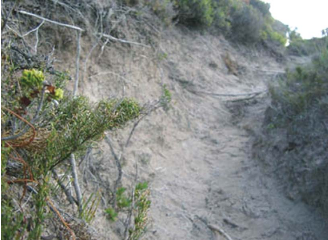
Figure 16 Bald Head trail PIN frame middle section showing a deeply incised trail set into a hillside, up-slope section to the left and an uncontained berm to the right which is leading to trail slumping on both sides as soil is moved along the trail centre (see Figure 12).
