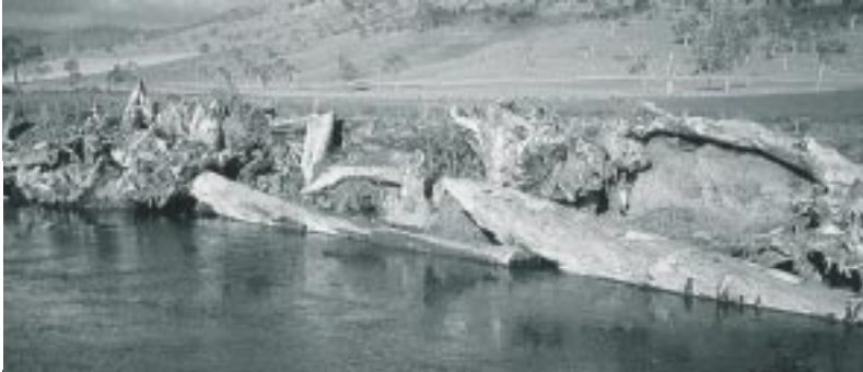
Logs and stumps used to stabilise banks.
