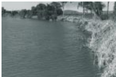
Eroded Stream Bank prior to construction of rock groynes.
