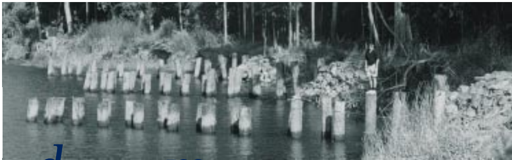
Below: Groynes on the Musgrave River, Old. Above: Pile groynes.
