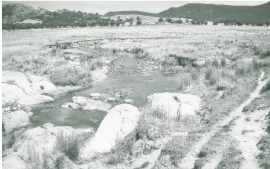
Actively eroding reach of Paddy's River with stock tracks, no native vegetation and uncontrolled stock access year round. The banks are further damaged by regular wombat holes. Algal blooms flourish here. Photo, Alison Elvin
