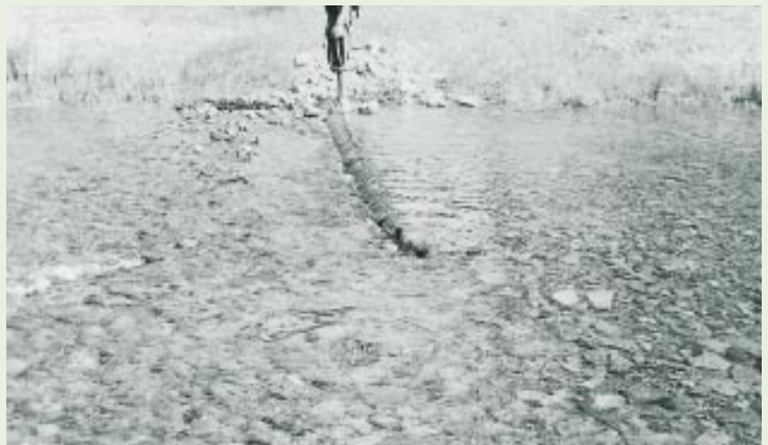
Photo 4: Cross-spanning LWD placed in the Pappinburra River, New South Wales. The structure has not been outflanked (yet) and has produced little associated bed scour.
