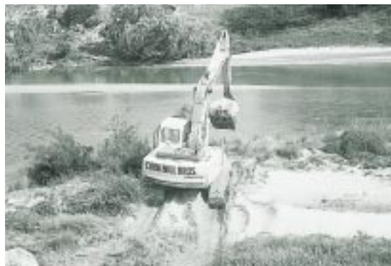
Left: Groyne 1 being installed.
