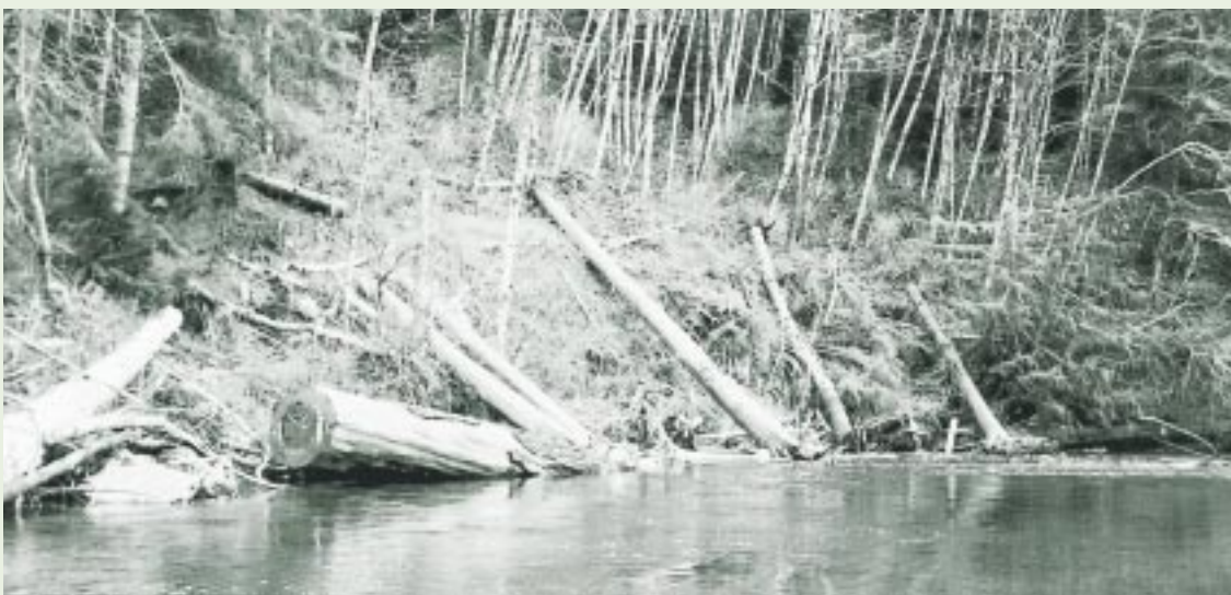
Photo 5: LWD with rock ballast was placed in Big Tree Creek, BC to dissipate stream energy and to deflect the thalweg (the line joining the deepest points of a stream channel) away from the outside bank. The root wads at the end of the LWD will increase the likelihood of pool formation and may also provide additional fish habitat. Flow is towards the bottom of the photo.
