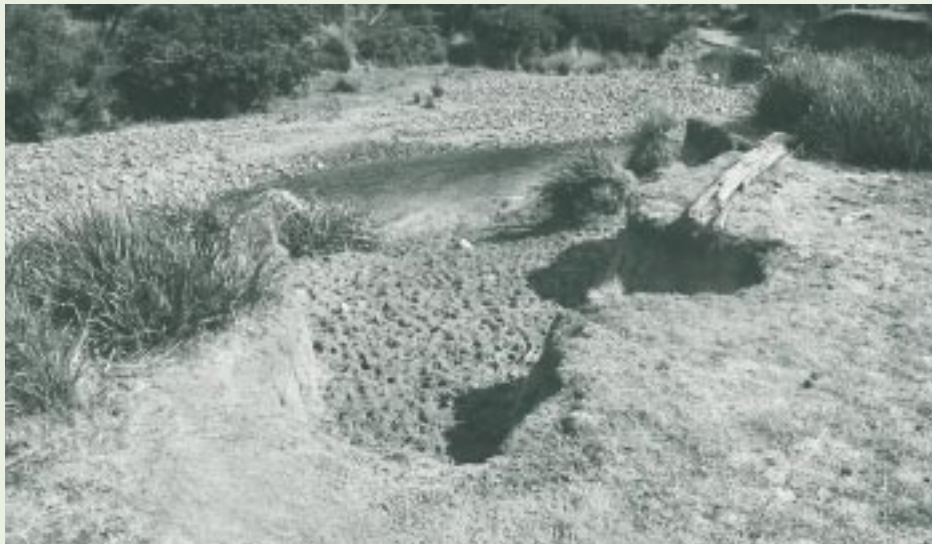
Unfenced Blackman River in Tasmania showing stock ramp pugging. Photo by Michael Askey-Doran.
