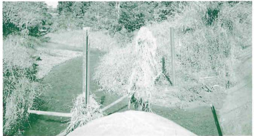
Top: Revegetation (right) protects creekbanks and steel posts (foreground) prevent flood-carried logs blocking culvert.
