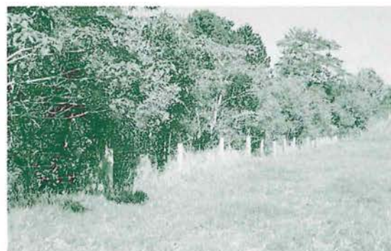
Top: Revegetation (right) protects creekbanks and steel posts (foreground) prevent flood-carried logs blocking culvert.
