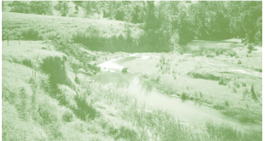
3: Before 1996, channel just starting to be constructed.
