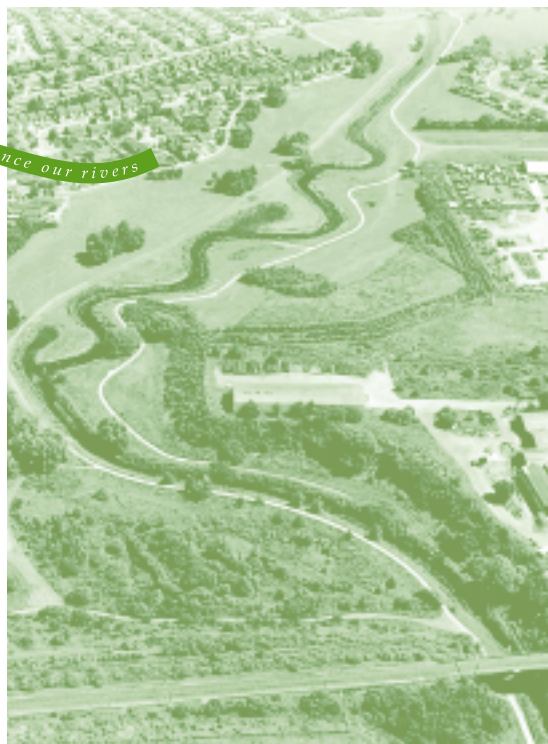
The River Skerne following restoration works
