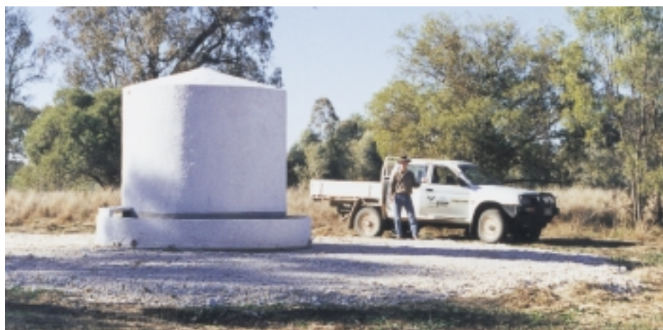
RiverReach on-ground works. Remote area watering system for seedling revegetation for the Moama Station revegetation project, north of Eulo and on Cookara Creek, tributary of the Paroo River. Generally revegetation is encouraged in semi-arid areas, however, in this situation revegetation will assist stabilisation of the creek bank, retard avulsion formation and reduce waterhole sedimentation.
