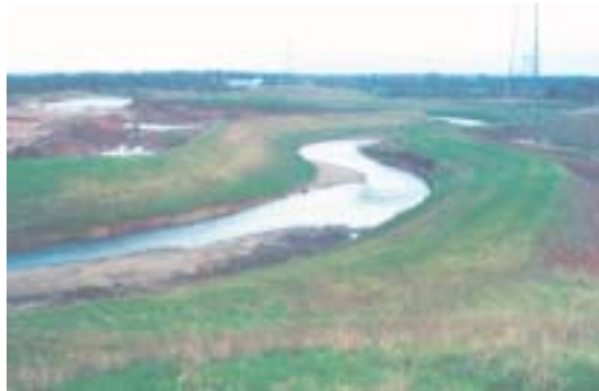
Left: River Tame M6 Motorway crossing, Birmingham Right: River Cole re-meandered reach, Birmingham
