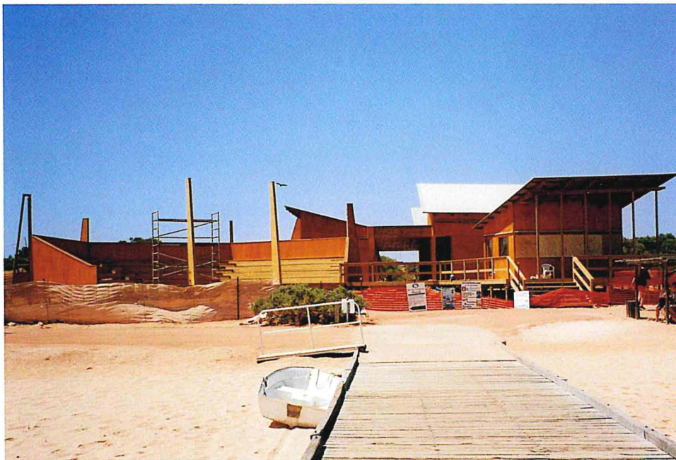
Under construction—the new Visitor Centre at Monkey Mia nears completion.
