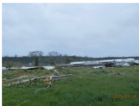
Poultry farm destroyed in Teoma, Efate Island, Shefa Province.
