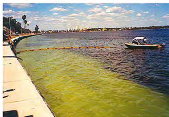
Using oil spill booms in Matilda Bay to concentrate and skim scums of Microcystis .
