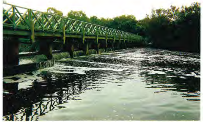
Figure 5: Water flowing over the Kent Street Weir at the beginning of the oxygenation season
