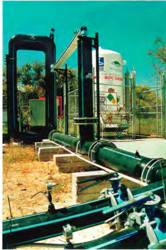
Figure 3: One of the two oxygenation plants used in the 1999/2000 project. Left: water pump in foreground with control panels and oxygen vessel behind. Right: Distribution pipes in foreground with oxygen dissolver and oxygen vessel in background
