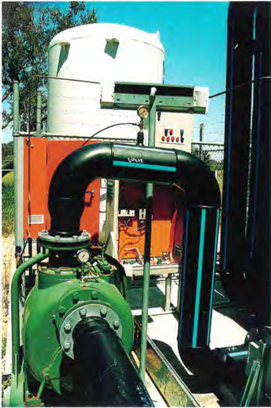
Figure 3: One of the two oxygenation plants used in the 1999/2000 project. Left: water pump in foreground with control panels and oxygen vessel behind. Right: Distribution pipes in foreground with oxygen dissolver and oxygen vessel in background
