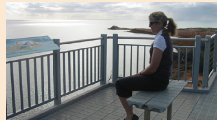
Shark Bay District PVS Coordinator Tricia Sprigg enjoys the view from the Eagle Bluff boardwalk in Shark Bay World Heritage Area. The deck, stanchions and seat top are all recycled plastic.
