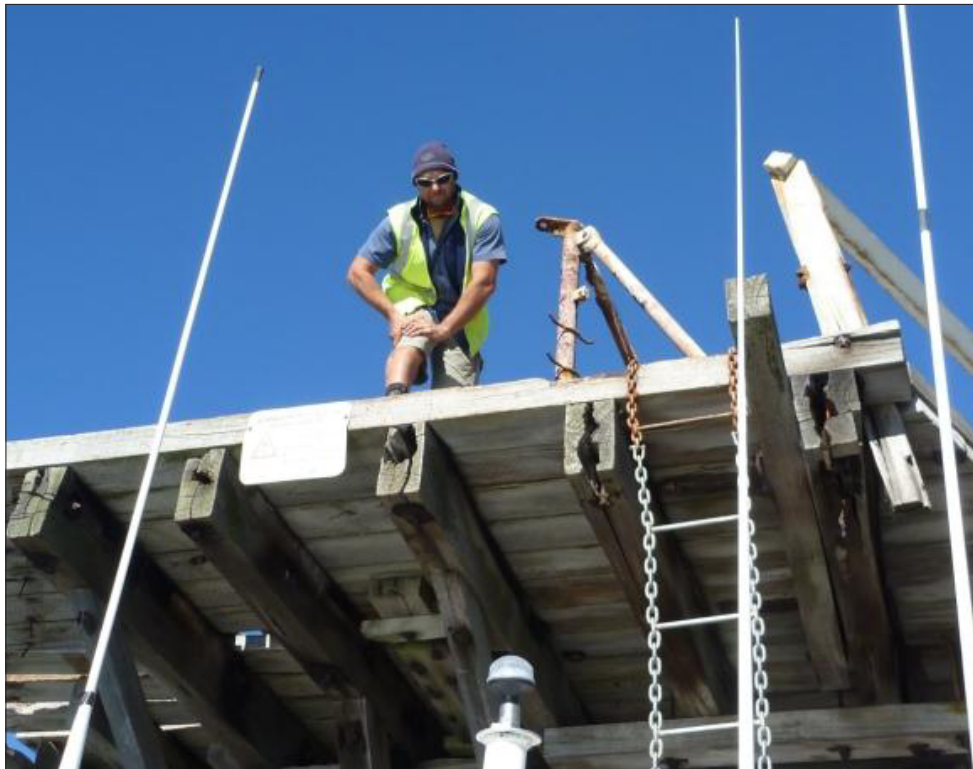
DEC site manager Rob Wilkes on the Breaksea Island jetty.
