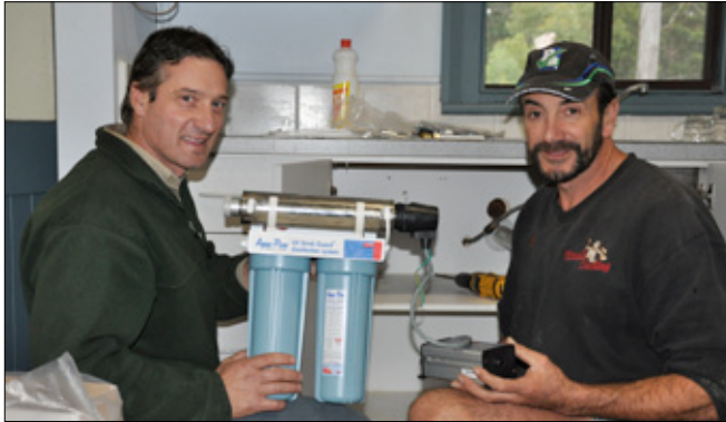
Project Manager David Favero (left) with the plumber installing a purifier.
