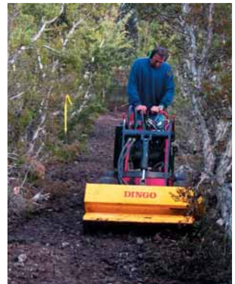
Rotary hoe process of lime application at eight tonne per hectare to trial rehabilitation of lands affected by acid sulfate soils. Photo – Alison Dugand
