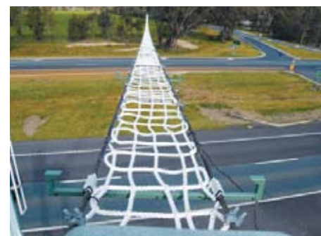
A rope bridge over the Hume Highway, Victoria, designed and installed by the Australian Research Centre for Urban Ecology (ACRUE, University of Melbourne) and VicRoads. Photo – Kylie Soanes (ACRUE) and Ross Meggs (Faunatech)
