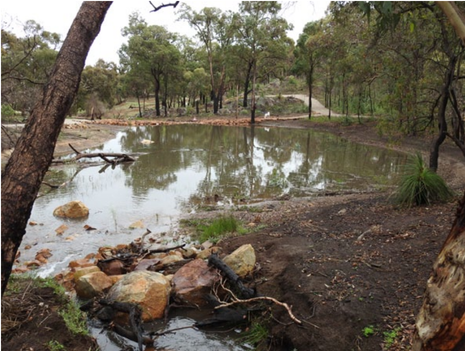
One of the two flowdams constructed to slow and hold water for short periods to combat stream erosion. You can also see the walk trail in the background. Photo – Mike Robinson.
