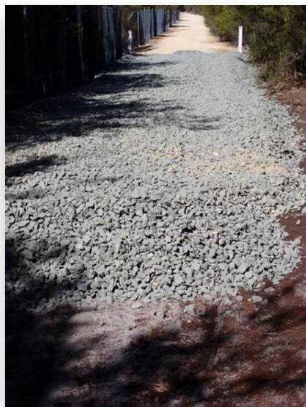
The limestone track and blue metal wash down bay help protect the spread of Phytophthora disease along tracks. It even works to some extent on preventing further disease spread by unauthorised off-road vehicles. Photo – Leonie Stubbs.
