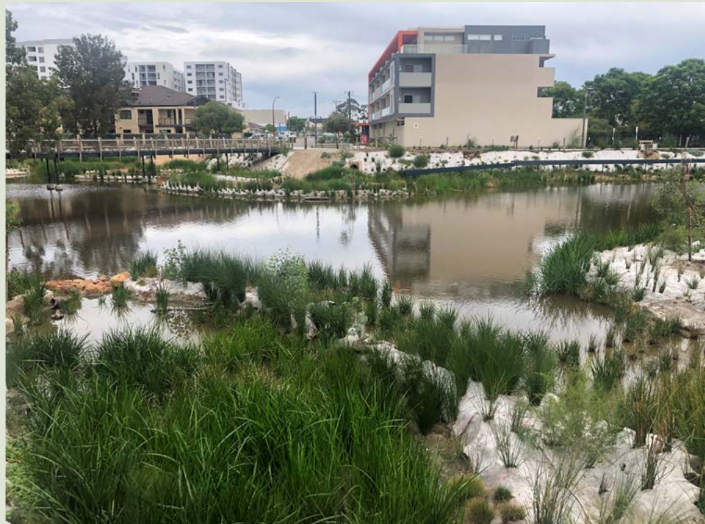
Wharf Street Basin in Cannington is a stormwater basin that has been redeveloped into a new public Next Generation Community Park, integrating landscape design and technology to create a space for people to relax in, a habitat for wildlife, and an education space, while still operating as a stormwater basin. Photo – Water Corporation.
